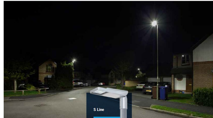
Street Lighting Installation Before and After
